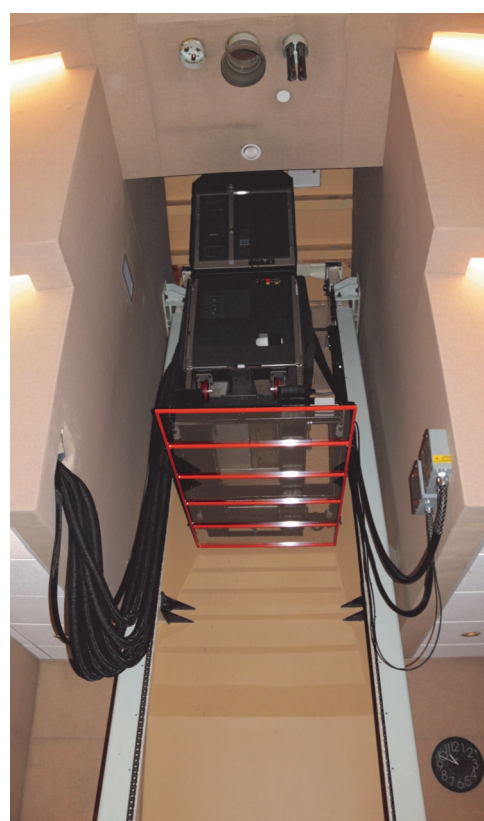
The IMAX with Laser projector installed in the Robert D. Lindner Family OMNIMAX Theater at the Cincinnati Museum Center in Ohio.
