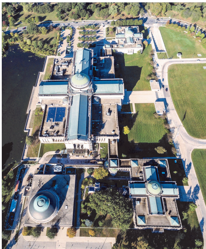
The Giant Dome Theater at the Museum of Science and Industry in Chicago has a D3D Cinema three-projector 6K laser dome system.
